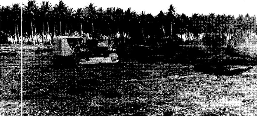
A major problem to be overcome before construction of the main airstrip at Cocos Island was the removal of wartime pierced steel planking. This was overcome by using a D-7 or D-8 tractor to cut it into 50 metre squares so that it could be rolled for ease of handling. (RAAF Museum)
